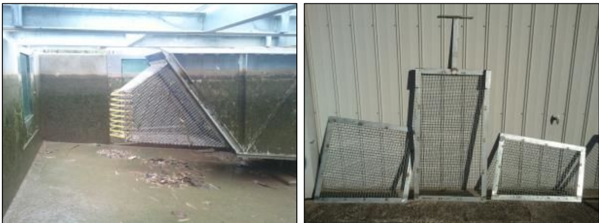
Figure 3.2: Left: Funnel on the exit of a Denil fishway in the Murray River, used to prevent fish from making return movements. Right: Screens to prevent fish escaping and trash from reaching the funnel.
