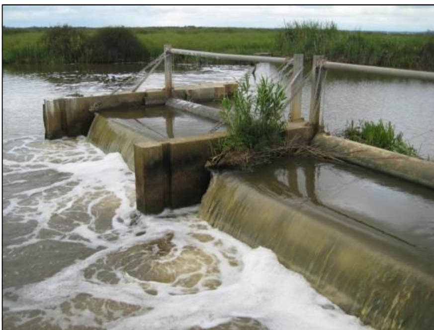
Figure 7. Tidal barrage gates on the Barwon River
