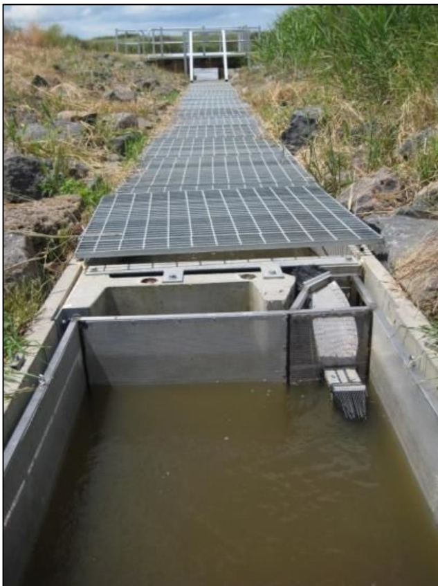
Figure 6. Barwon River vertical-slot fishway with fishway exit trap shown in position.
