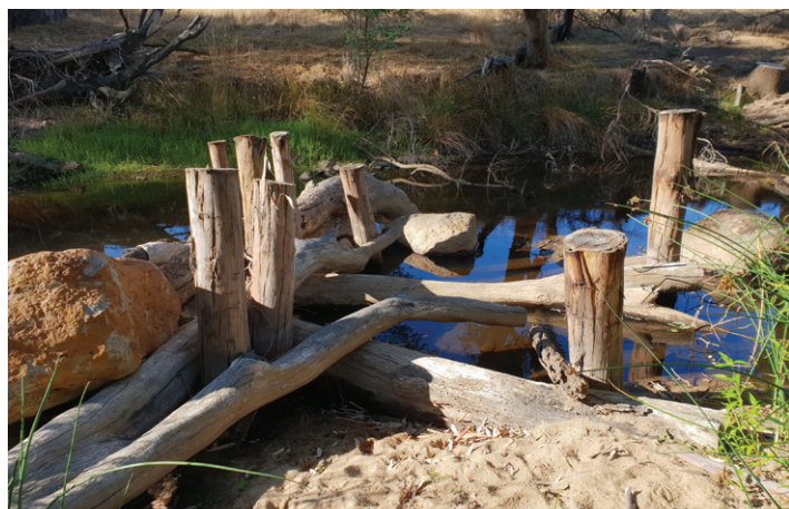
Hughes Creek instream woody habitat structure: timber pieces are keyed into the riverbank, locked into one another, and secured using piles and rocks. (Photograph: Renae Ayres, ARI)
