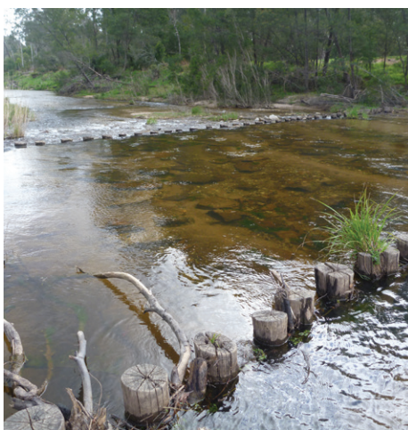
In the Cann River, multiple timber piles are embedded across the waterway channel to slow the movement of the sandy substrate. (Photograph: Renae Ayres, ARI)
