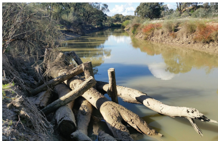
Timber structure installed in Pyramid Creek, consisting of two rootballs and four lengths of timber, pinned to the substrate with 8-10 timber piles. (Photograph: North Central CMA)
