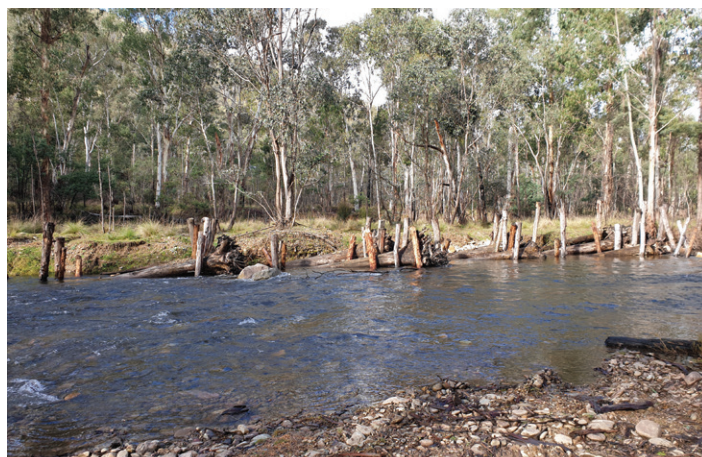
Macalister River instream woody habitat structures involving a series of rootballs with tree trunks, pinned together and anchored by timber piles. (Photograph: Renae Ayres, ARI)
