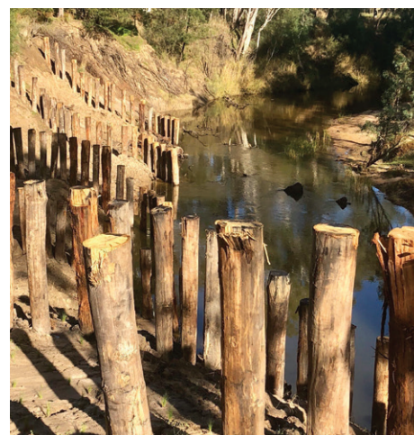
Timber piles are pinned vertically into the edge of the river channel to mitigate erosion. (Photograph: Glenelg Hopkins CMA)
