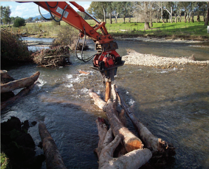
Timber structures may be anchored and stabilised using materials such as timber piles, cables, rocks, anchors and concrete. (Photograph: Goulburn Broken CMA)
