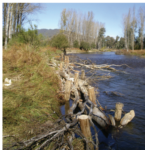
Tree trunks and branches are pinned together to create instream woody habitat structures in Narie Creek (Photograph: North East CMA)
