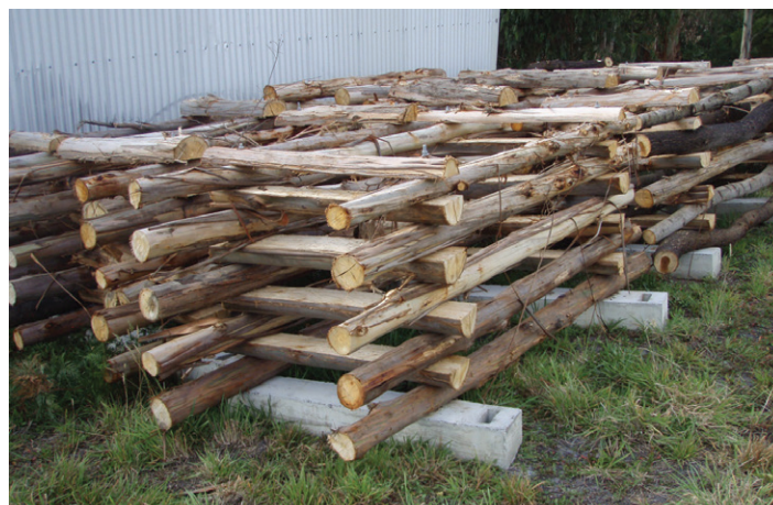
'Fish havens' or 'fish hotels' consist of many relatively small branches arranged in a square or rectangular shape. They are connected by metal rods, and sometimes weighted with concrete and pinned with piles. (Photograph: Corangamite CMA)
