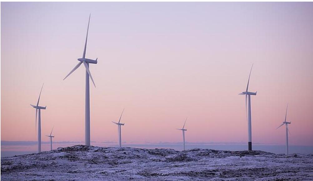
**Figure 7. Smøla vindpark, showing snowy conditions and a turbine (right) painted at the base to reduce collisions for Willow ptarmigan. Source: Emelysjosasen, CC BY-SA 4.0.**
