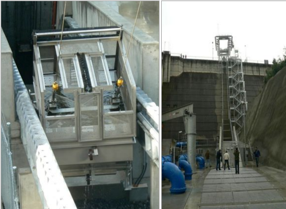
Figure S18. Fish lift constructed at Tallowa Dam on the coastal Shoalhaven River in south-eastern NSW. The ascending hopper is shown on the right (photos: Janet Pritchard).
