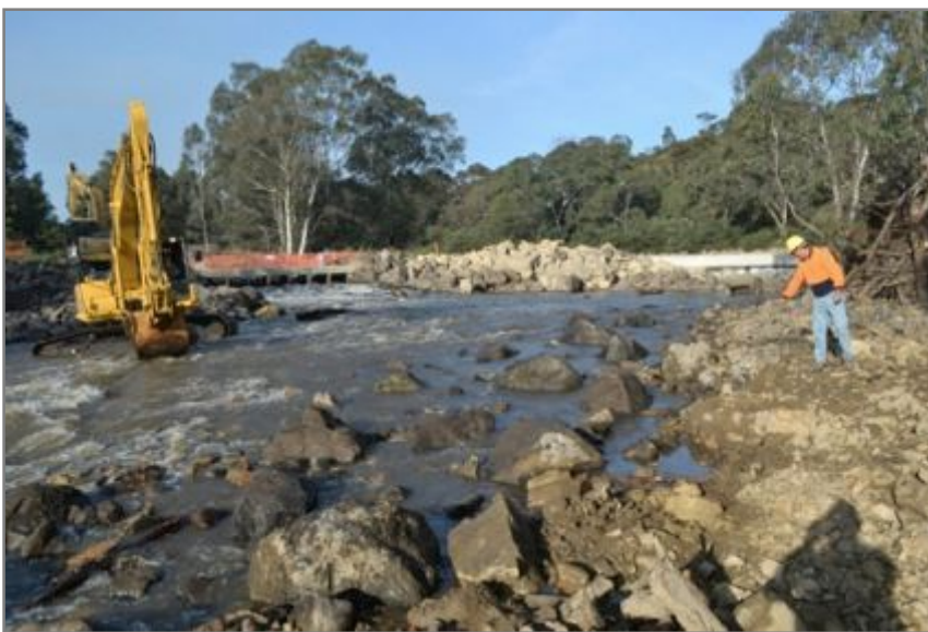
Figure S14. The full-river-width random-rock fishway on the coastal Yarra River at Dights Falls (Melbourne) in 2012. Note that the rocks are placed to maximise the edge effects of the bank and provide fish with a continuous path of ascent (photo: I. Stuart).
