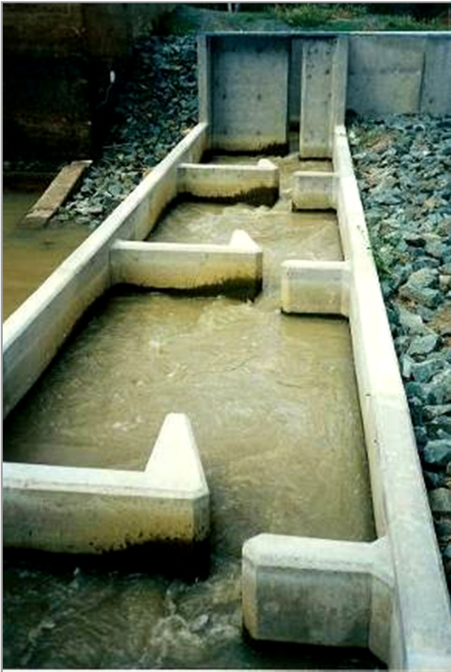
Figure S2. A vertical-slot fishway on Broken Creek in northern Victoria. Note the low pool turbulence and water velocities (photo: I. Stuart).
