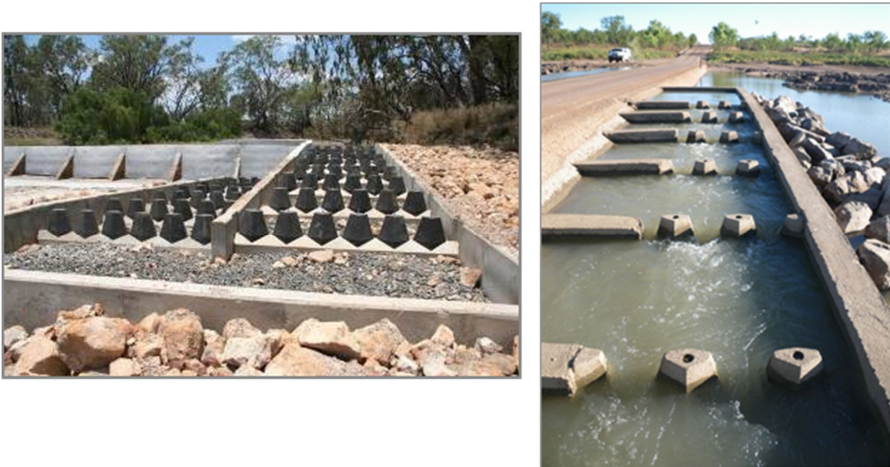
Figure S8. (Left) Pre-cast plastic cones and (right) concrete cones, which break up laminar flow and provide roughness for fish to ascend culverts in Qld (photos: A. Berghuis and T. Marsden).
