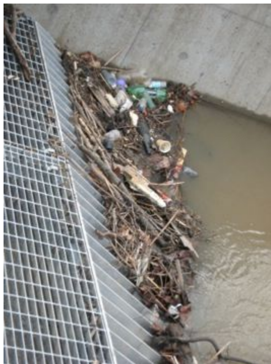
Figure 15. Regular clearing of trash racks is required to maintain attraction flows into fishways and to maintain appropriate head loss (and therefore velocities) at the exit.
