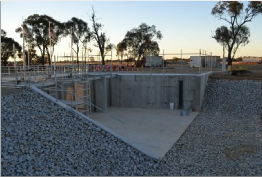
Figure S16. The Hipwell Offtake regulator on Gunbower Creek nears completion in November 2013. This structure includes a fish lock, with the entrance slot noticeable on the right side of the picture (photo: I. Stuart).
