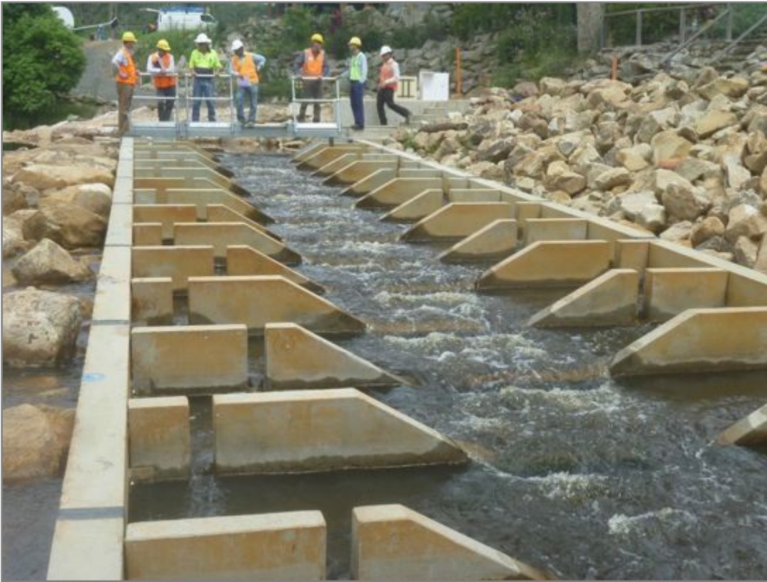
Figure S9. A trapezoidal fishway on the coastal Wyong River in central NSW. This type of innovative fishway is still subject to evaluation, but appears to have strong application and will also be trialled at the Murray River barrages located near the Murray River mouth from 2015 (photo: M. Mallen-Cooper). One interesting aspect is the splash zone at the edges of the trapezoidal weirs, which may facilitate the passage of climbing fishes.
