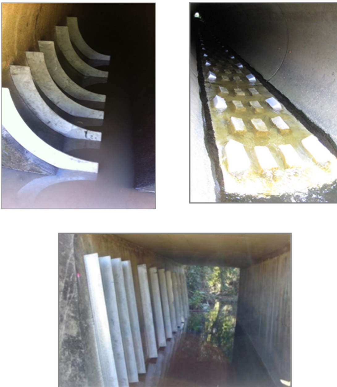
Figure S11. Some options for improving fish passage at existing culverts. (Top left) Pipe, (top right) spoiler baffles and (bottom) box culverts with retrofitted one-side baffles. Baffles help to slow water velocity and create eddies for fish to rest in during their upstream migration. The pipe culvert baffles (top left) are newly installed on Cardinia Creek in eastern Melbourne, along with a rock fishway. Photos: courtesy T. Marsden and Melbourne Water.
