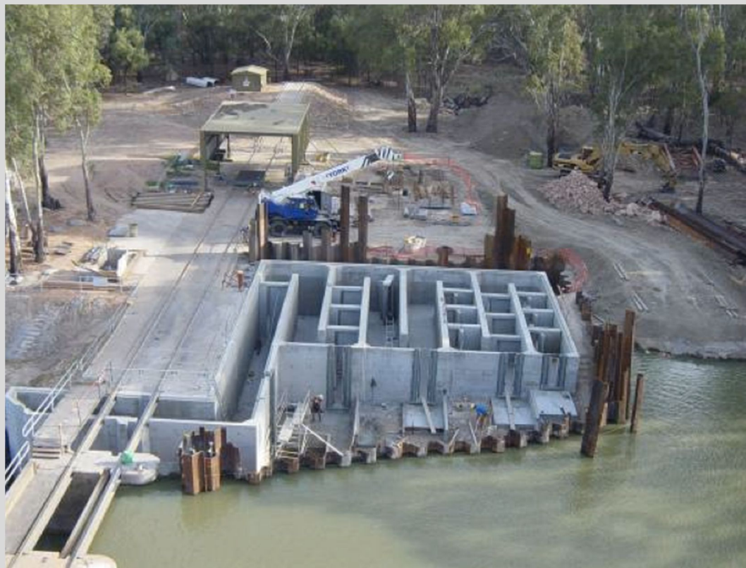
Figure B3.1. Vertical-slot fishway under construction at Lock 9 in 2005 (photo: A. Richter).
