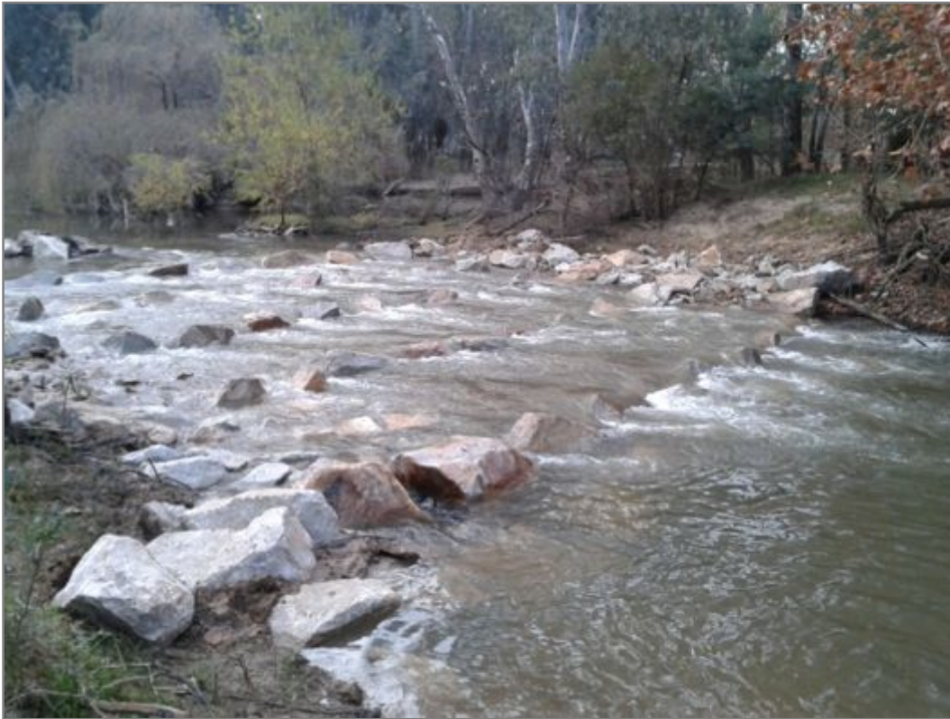
Figure S15. The upper leg of the Wangaratta rock-ramp fishway on the Ovens River in 2010. Note the raised rocks on the bank margins that increase the headwater range of the fishway (photo: T. Marsden).
