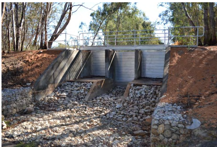
Figure 7. The Little Lake Hattah regulator, where Carp screens for subadult and adult fish were installed in 2013
