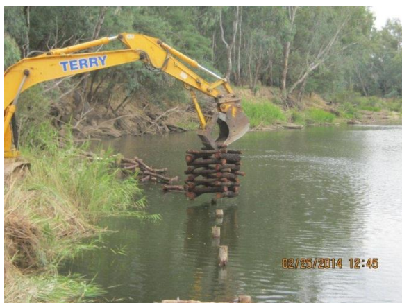
Placing fish hotels (structural habitat) into the Ovens River. Photo: A. Wilson
