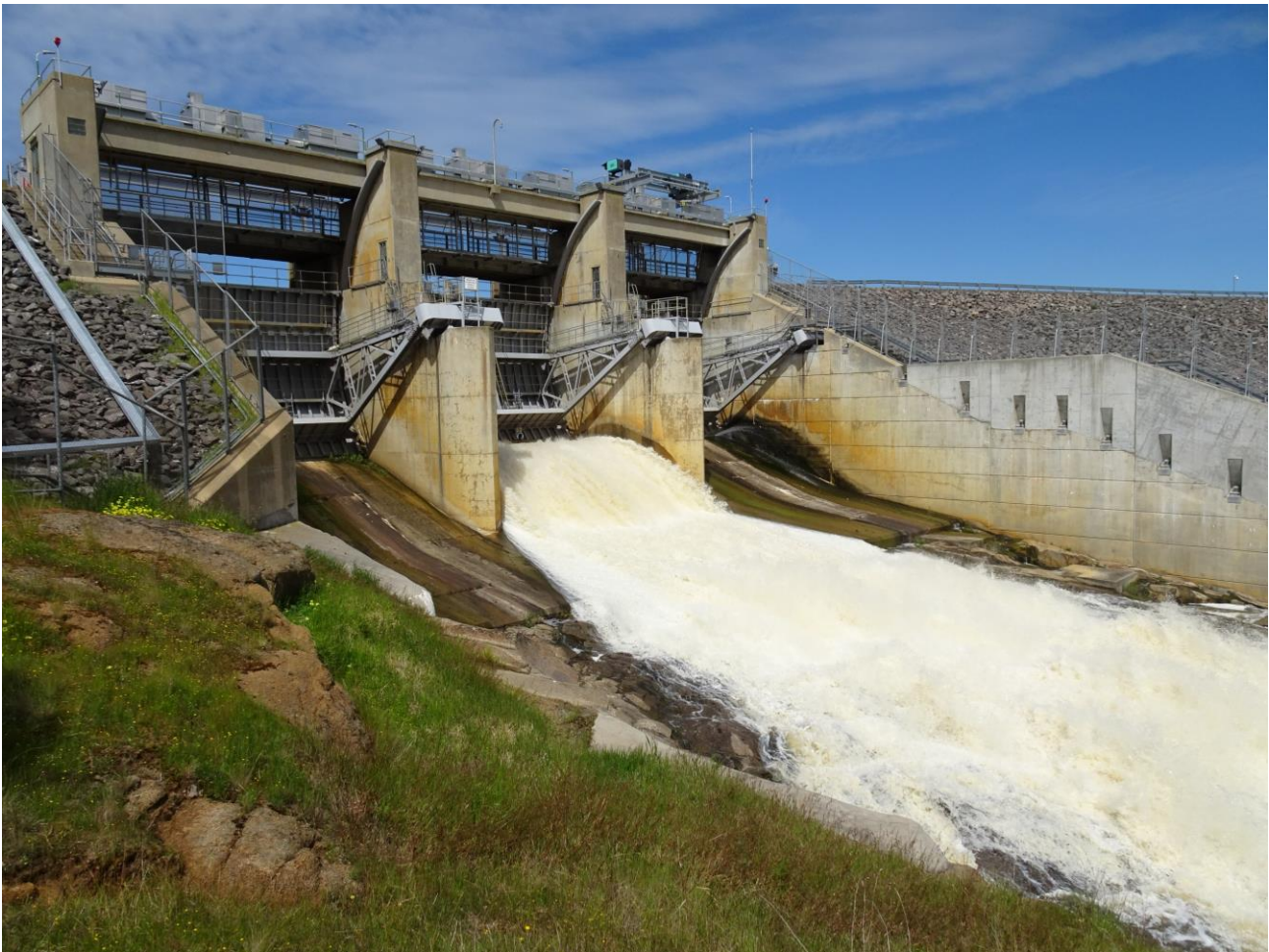
Figure 8. Water being released from Cairn Curran Reservoir via a controlled (gated) spillway
