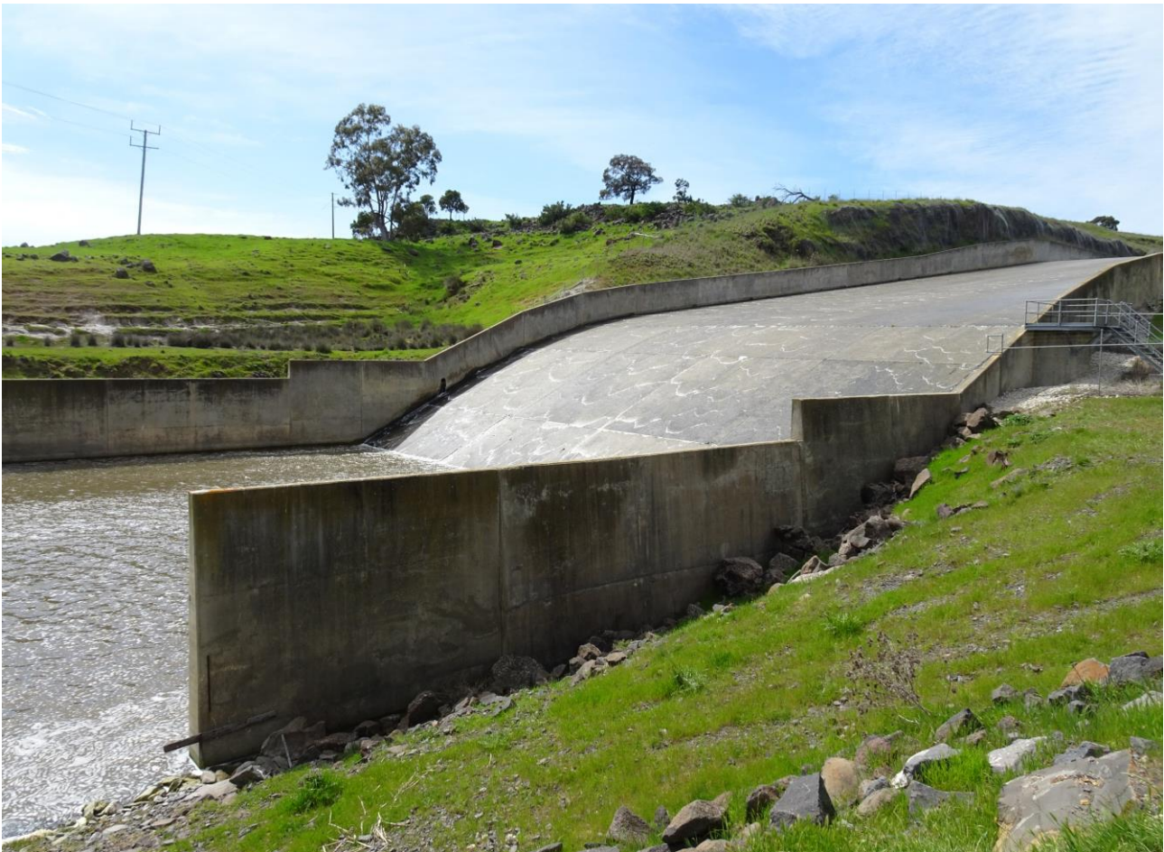
Figure 11. The outer edge of the spillway wall at Tullaroop Reservoir
