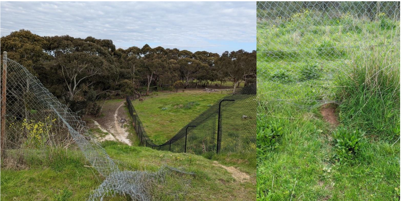
Figure A9. Fencing around Kelynack Dam (left), showing animal path evident under one fence (right)
