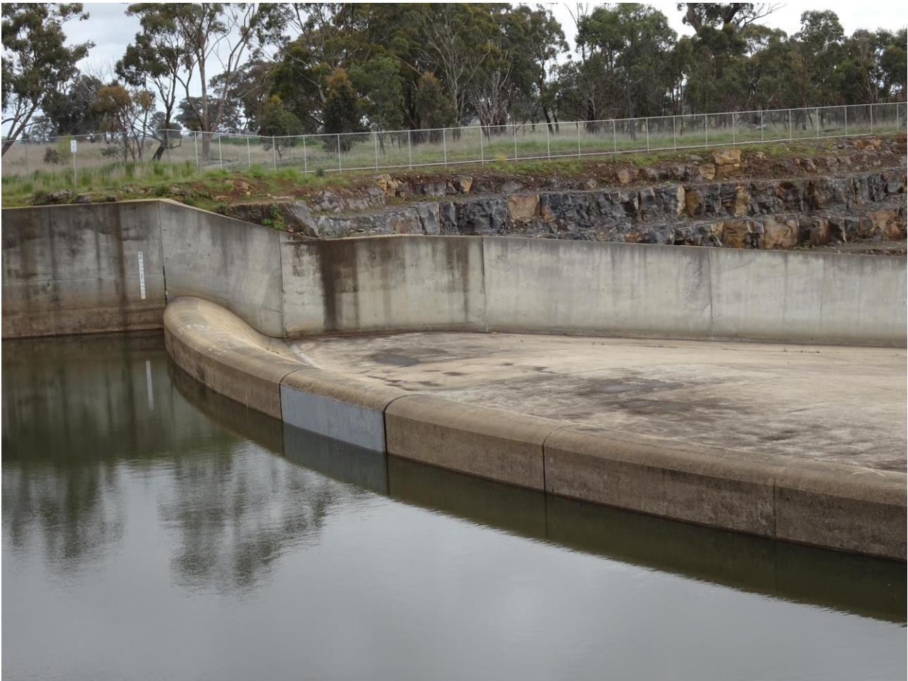
Figure 5. Lake Eppalock spillway crest, viewed from the weir pool end
