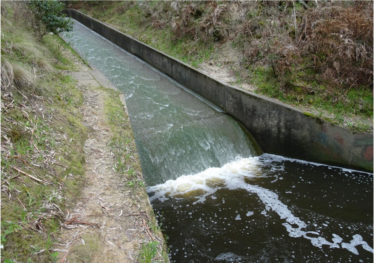
Figure 7. Steeply sloping spillway surface at Gong Gong Reservoir, viewed from the downstream end
