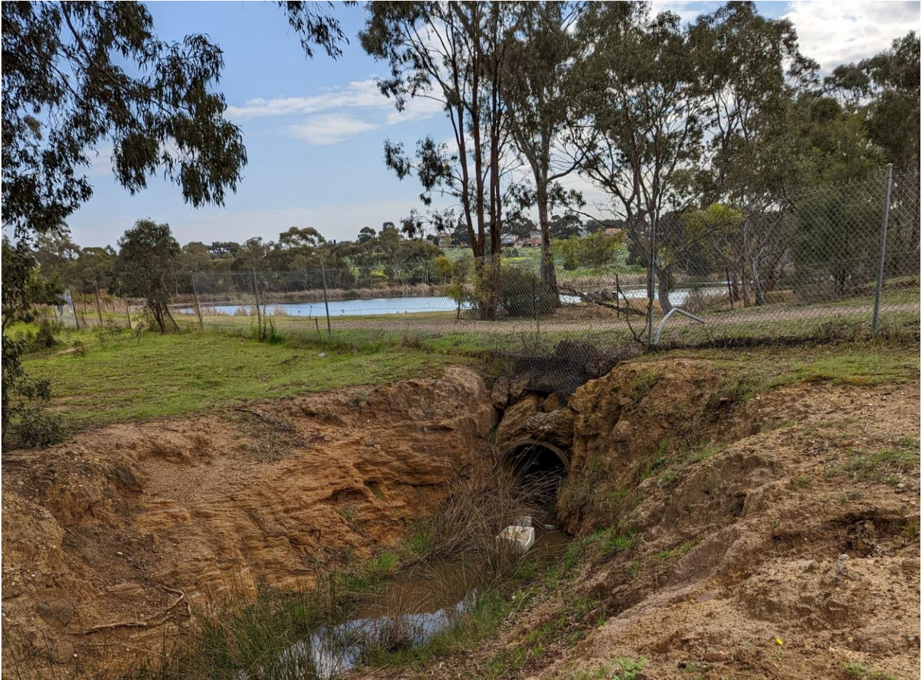
Figure A8. Culvert emerging from lower end of Kelynack Dam, showing some water pooling near the outlet
