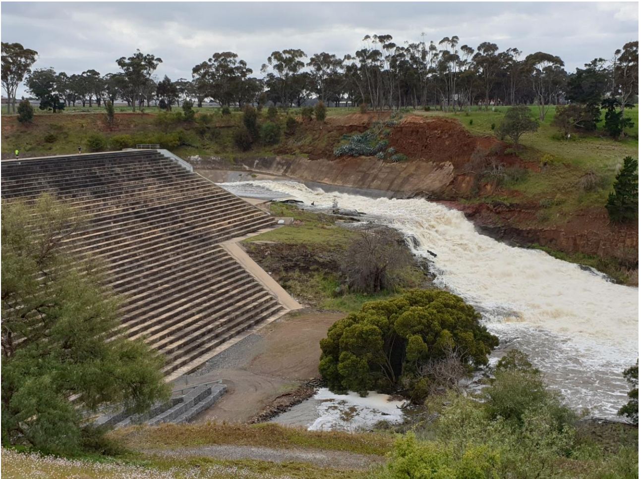
Figure A3. Melton Dam in high flow in September 2022, showing stepped wall and spillway
