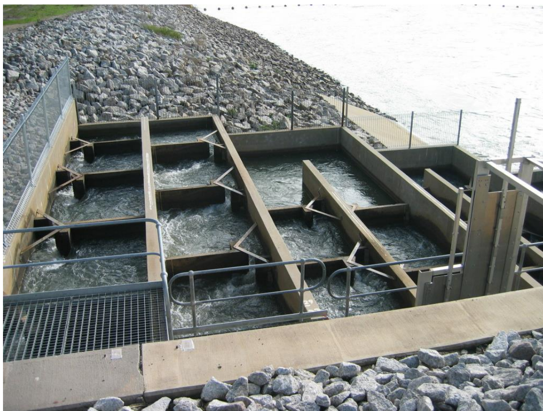
Figure 3. A vertical-slot fishway designed for movement of medium- to large-sized fish presumably should also be navigable by a platypus
