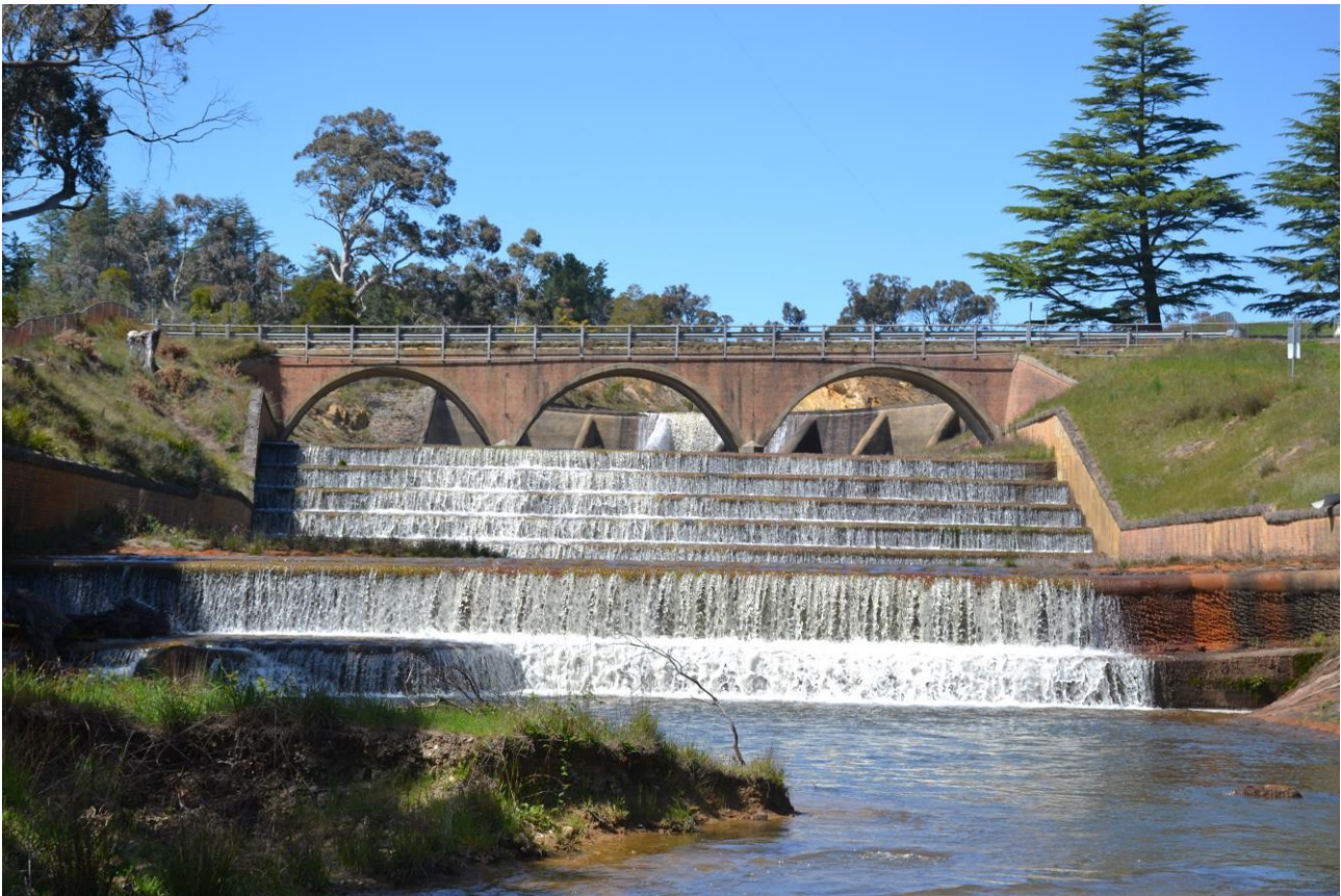
Figure 6. Stepped spillway at Upper Coliban Reservoir, viewed from the downstream end
