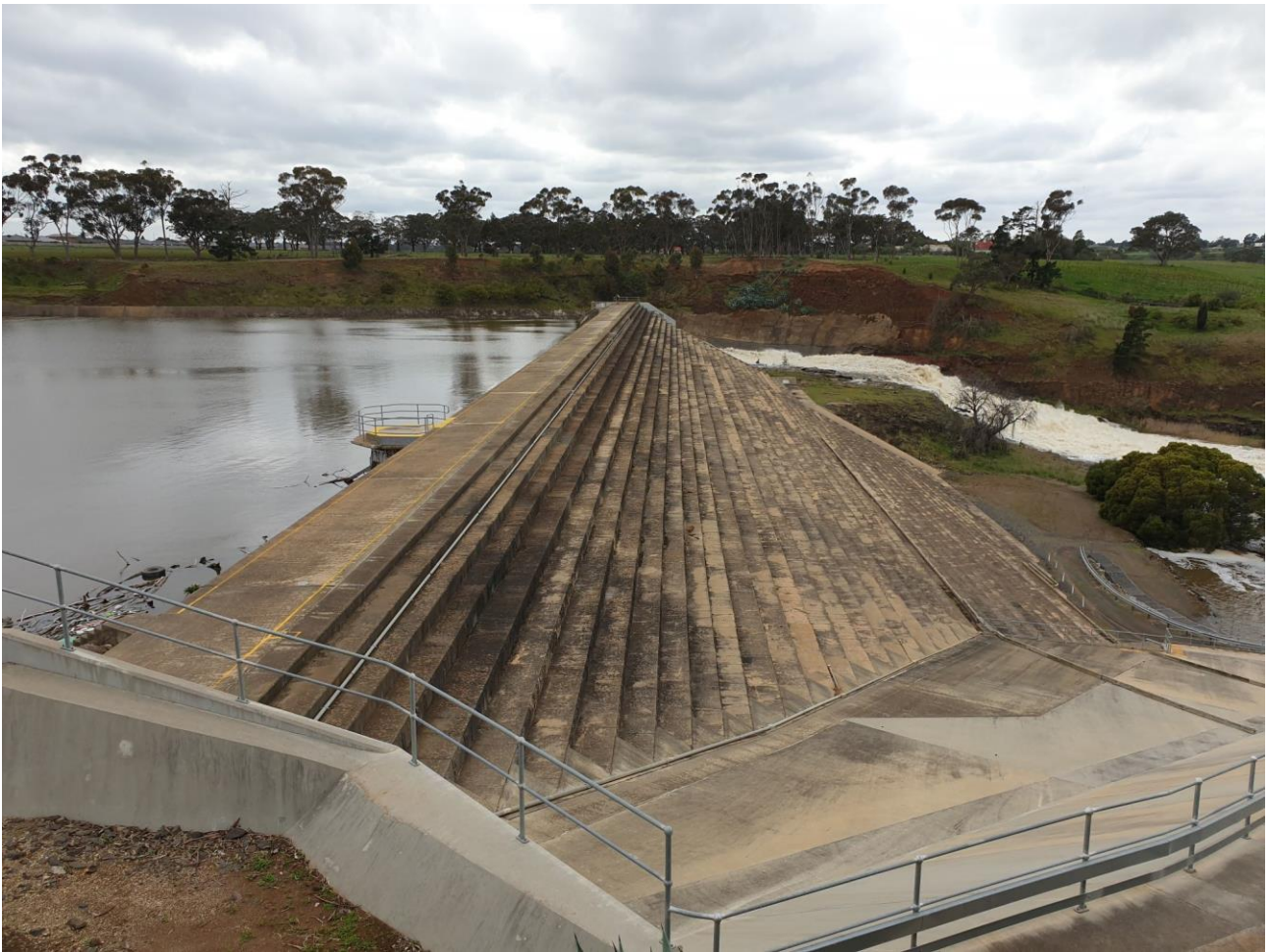
Figure A4. Melton Dam showing stepped wall with surrounding extensive concreted areas
