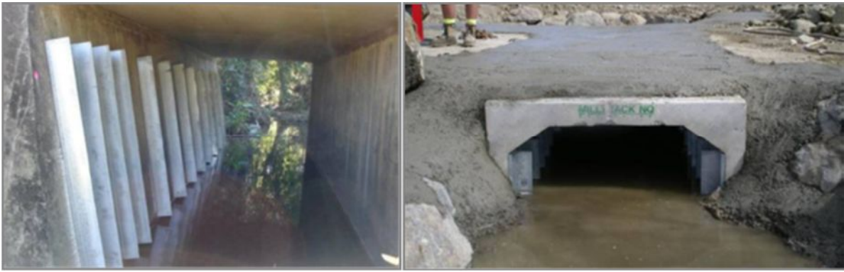
Figure 3.3: (Left) Box culverts with retro-fitted one-side baffles and (right) twin-sided baffles. Baffles help to slow water velocity and create eddies for fish to rest in during their migration. (Photos courtesy Tim Marsden.)
