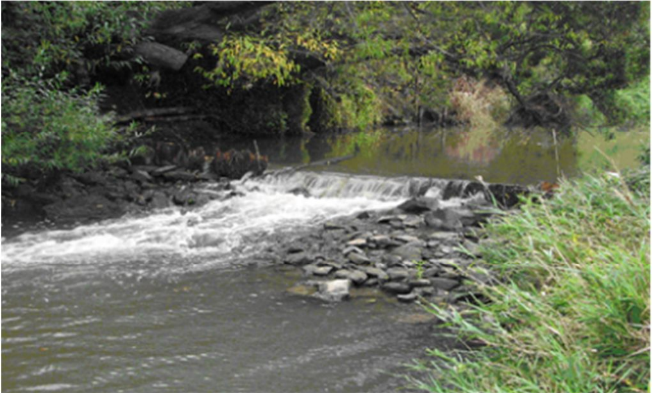
Figure 2.5: A fixed crest sheet pile gauging weir with excessive downstream water velocity, head loss and turbulence, which severely impedes fish migration.
