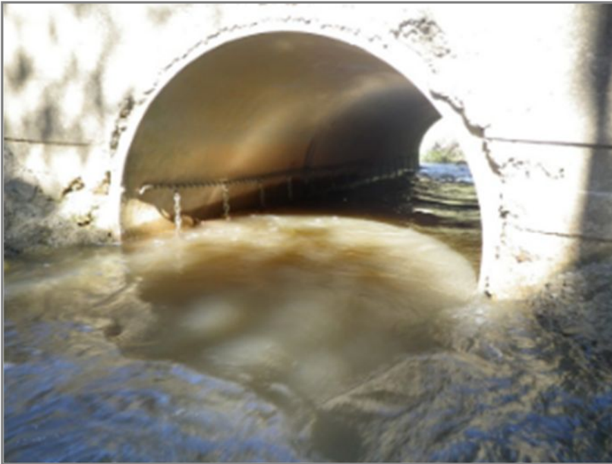
Figure 3.8: Chain with droppers facilitates small-bodied fish migration through pipe culverts in Queensland. Chain droppers and mussel spat ropes can be considered experimental low-cost fish passage options that require further field evaluation. (Photo courtesy Tim Marsden.)
