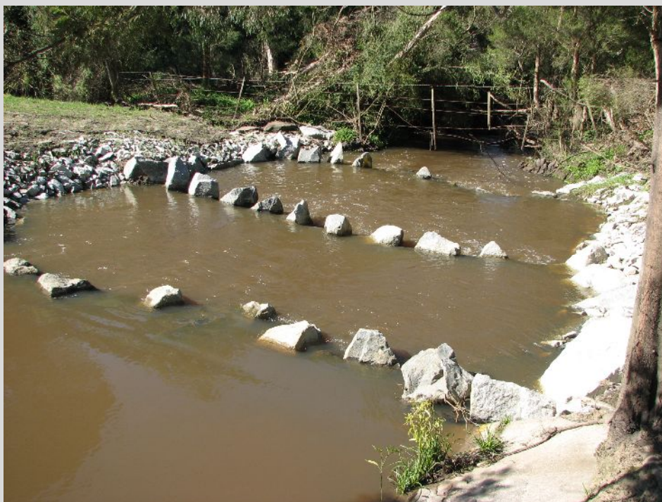
Figure B3.1: Cardinia Creek lateral ridge rock-ramp fishway
