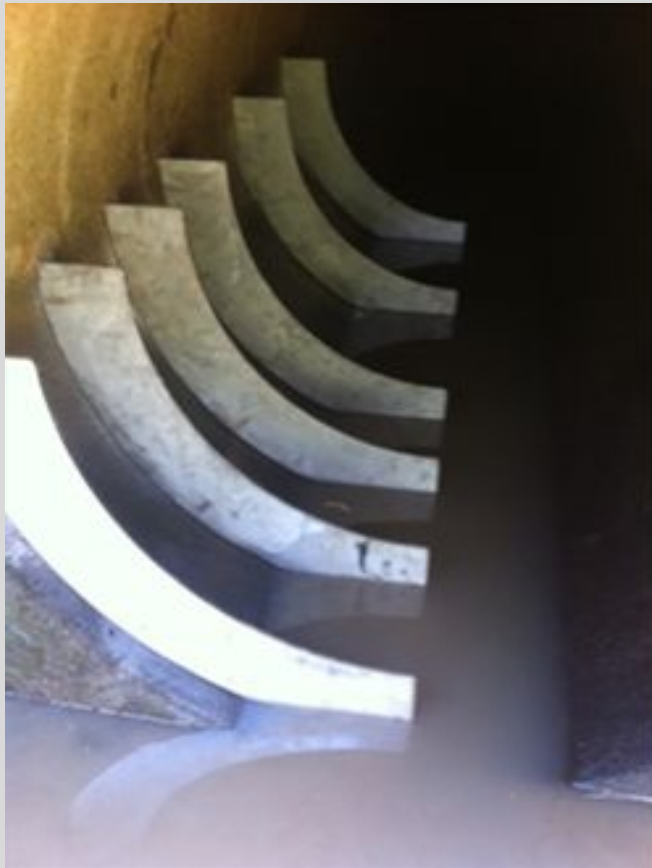
Figure B3.2: Cardinia Creek culvert baffles.
