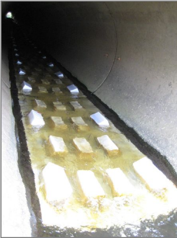
Figure 3.7: Spoiler baffles which break up laminar flow and provide roughness for galaxiids to ascend culverts in New Zealand. These have proven successful in short culverts (e.g. 6 m long) but unsuccessful in long culverts (e.g. 70 m long).
