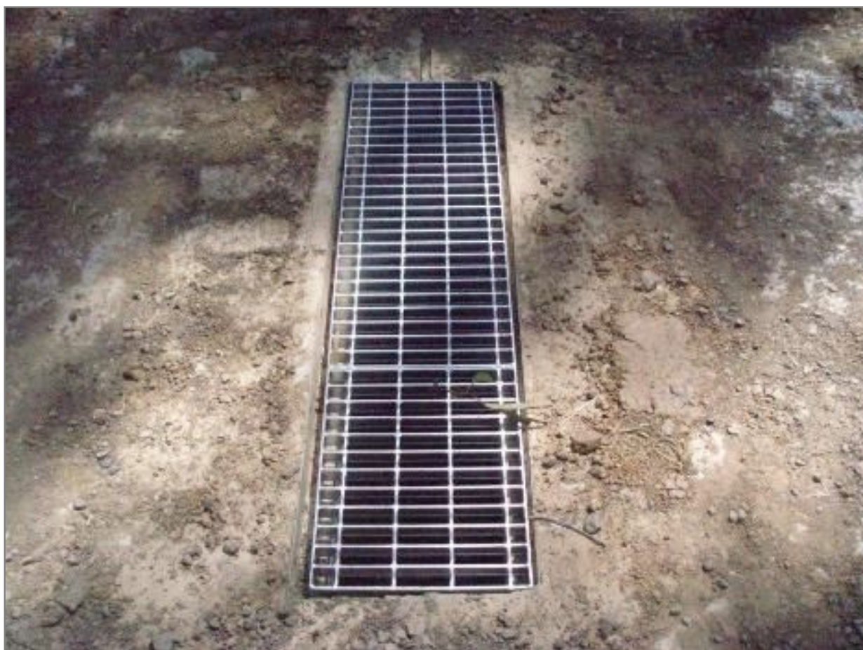
Figure 3.1: A light grid in a new wetland culvert to facilitate passage of native fish.
