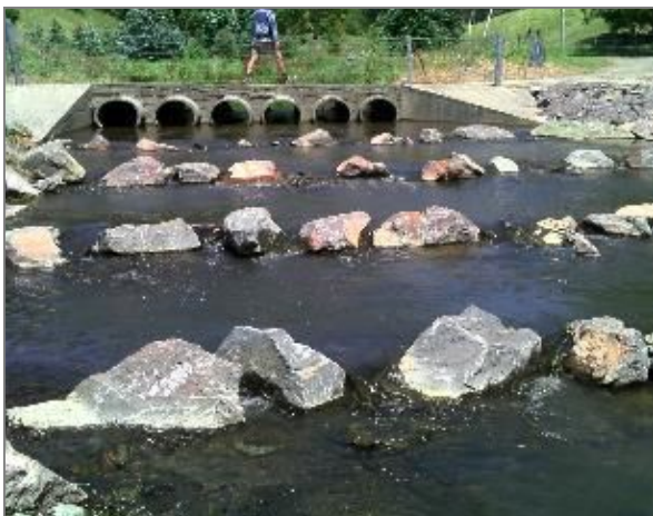
Figure 3.9: Some recent rock fishways which back up water through culverts to create low water velocity for passage of small-bodied fish. This type of approach can be expensive but is cost-effective at high priority sites for existing culverts.
