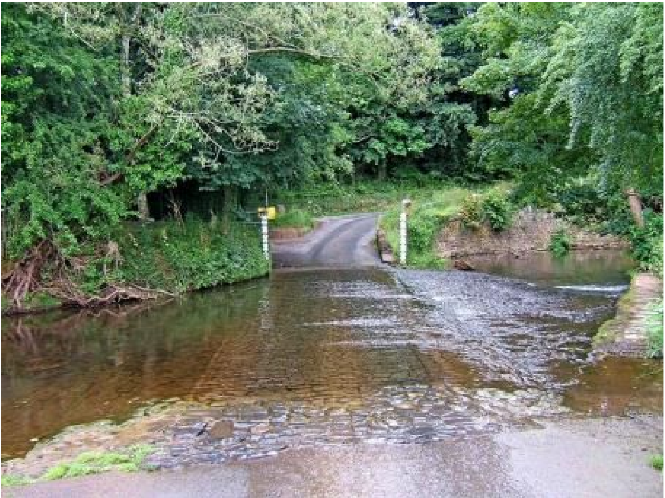
Figure 2.4: Ford crossing with shallow depth and streaming laminar flows that severely affect fish migration.
