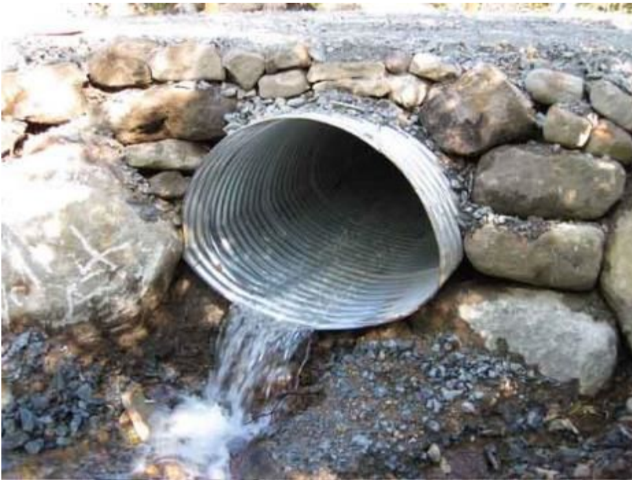
Figure 2.1: Erosion at the downstream end of culverts can result in considerable head loss (i.e. culvert perching) and consequent barriers to fish movement.
