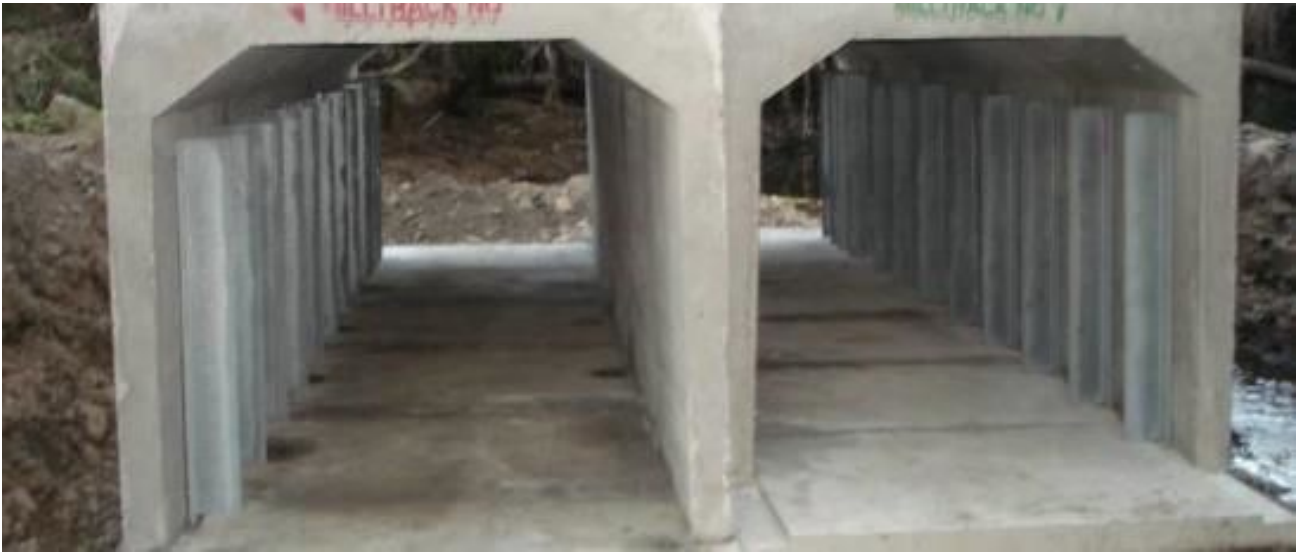
Figure 3.5: Box culverts fitted with single-sided baffles.
