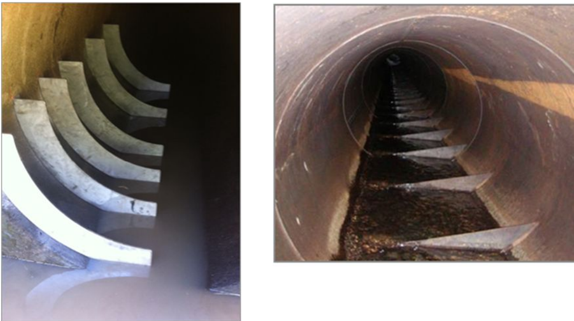
Figure 3.4: Pipe culverts fitted with single sided baffles.
