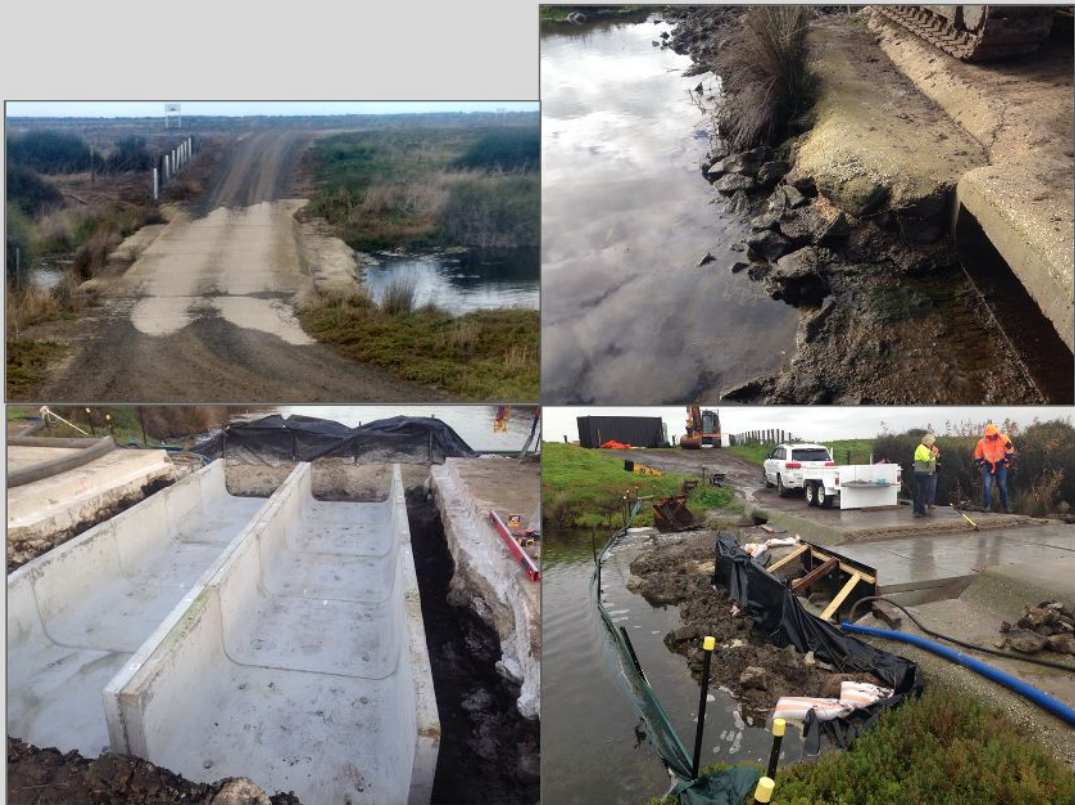
Figure B2. On the Little River, in coastal Victoria, Melbourne Water replaced a single perched culvert (top left and right) with a paired optimised culvert (bottom right and left). Note that the upstream and downstream invert of the new culverts are 0.3 m below bed level, there is a flat culvert slope and zero water velocity. (Photos courtesy of Melbourne Water.)
