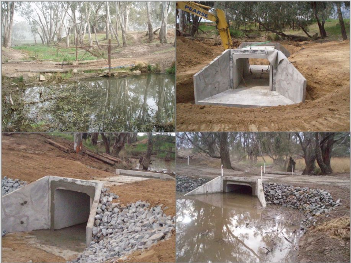
Figure B1: Replacement of a submerged pipe culvert (top left) with an optimised box culvert (top right and bottom). Note that the upstream and downstream invert of the box culvert is below bed level, there is a flat culvert slope, no water velocity and the high sides of the culvert maximise light penetration. (Photos courtesy of Goulburn Broken CMA.)
