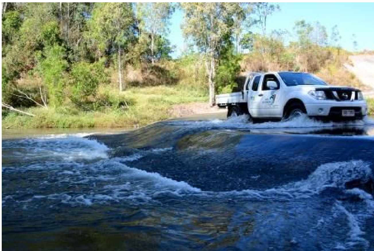
Figure 2.3: Road causeway with shallow depth, high (e.g. 1 m) total head loss and streaming laminar flows that severely impacts on fish migration.
