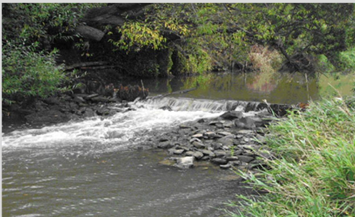
Figure B4.1: The Tarwin River Weir showing the stepped sheet pile structure and erosion control rock.
