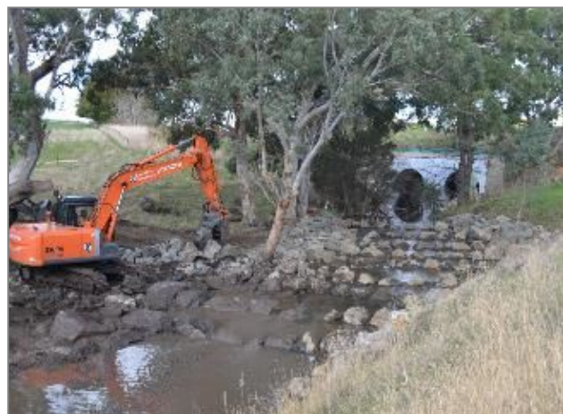
Figure 3.9: Some recent rock fishways which back up water through culverts to create low water velocity for passage of small-bodied fish. This type of approach can be expensive but is cost-effective at high priority sites for existing culverts.
