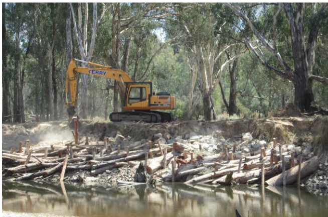
Using wood to protect banks on the Ovens River
