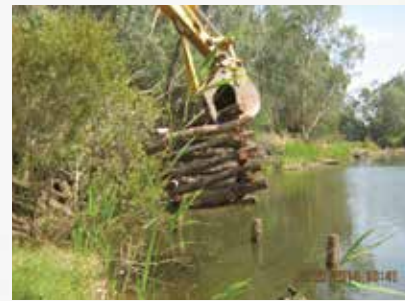
Fish hotel being put in place
