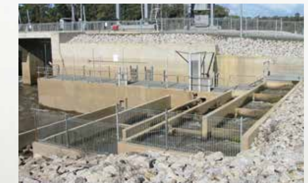
Torrumbarry vertical slot fishway
