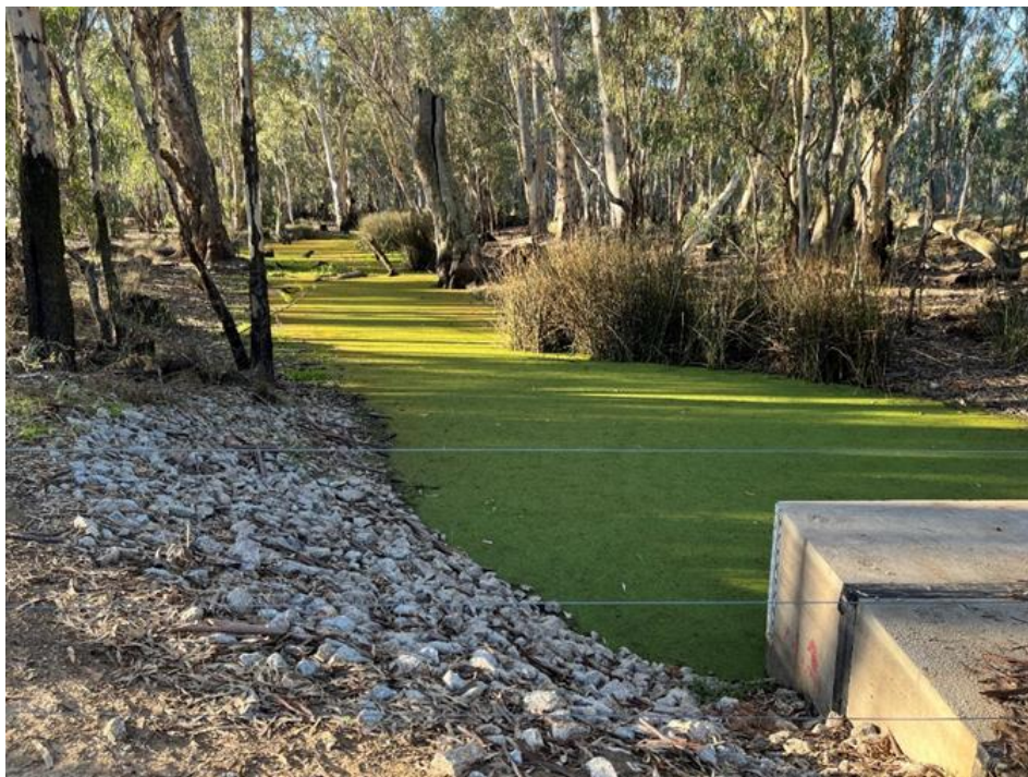
Figure 3. Example of the leaky regulator concept at Reedy Lagoon in September 2023. The photo shows the habitat provided by 'leaking' water from the regulator (shown bottom right) into the channel connecting the Gunbower Creek with Reedy Lagoon. This photo was taken following extensive flooding in 2022, which caused the growth of surface-dwelling aquatic plants that degraded the usually diverse aquatic vegetation at the site.
