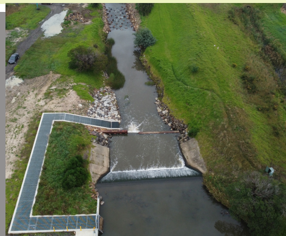
An aerial shot of Pillars Crossing on Dandenong Creek, showing a cone fishway and rock ramp fishway (Credit: Danial Robbins, Melbourne Water)
